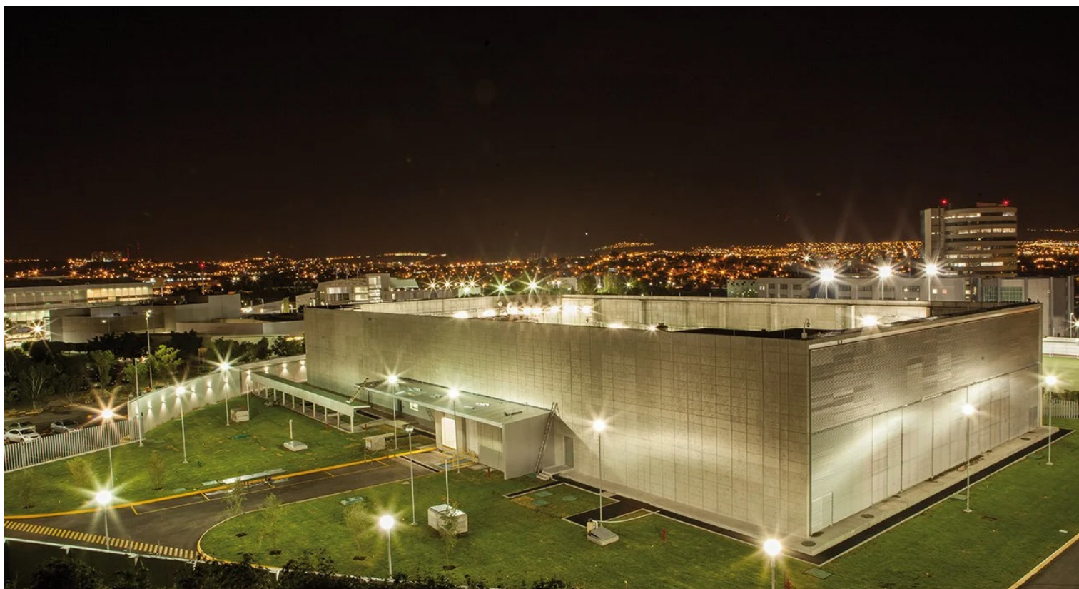
Project Q data centre - Lorong Chuan, Singapore
